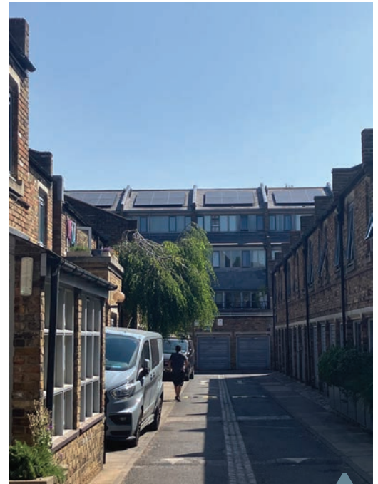
SOLAR PANELS on the roofs at Pugin Court
