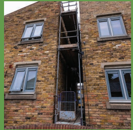
Homes at Barnsbury Mews have now been retrofitted.
