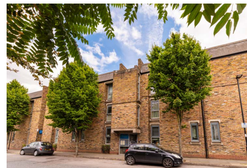
Solar and heat pumps for Pugin Court
