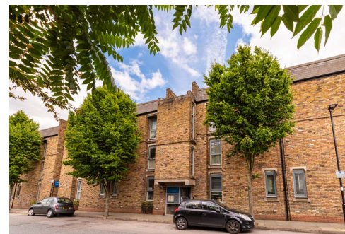
Solar and heat pumps for Pugin Court
