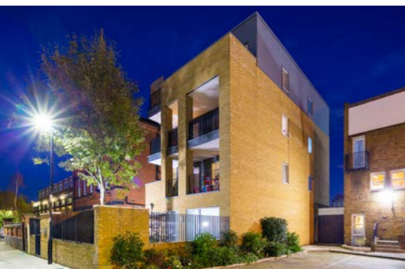
Eden Grove's living rooms open onto balconies, giving better natural lighting and ventilation and letting tenants enjoy the mature tree that was retained on site
