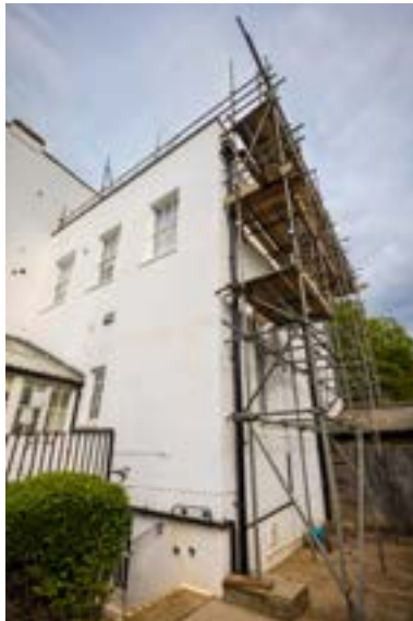
A large portion of our repairs budget went on roof repairs last year following repeated downpours caused by our changing climate
